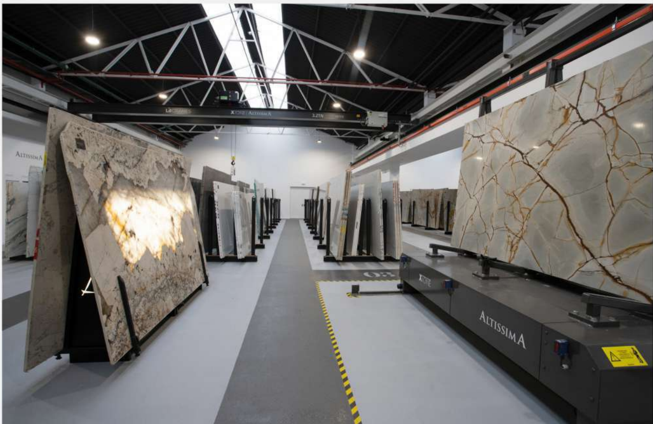
3.2Tn double girder overhead crane installation
