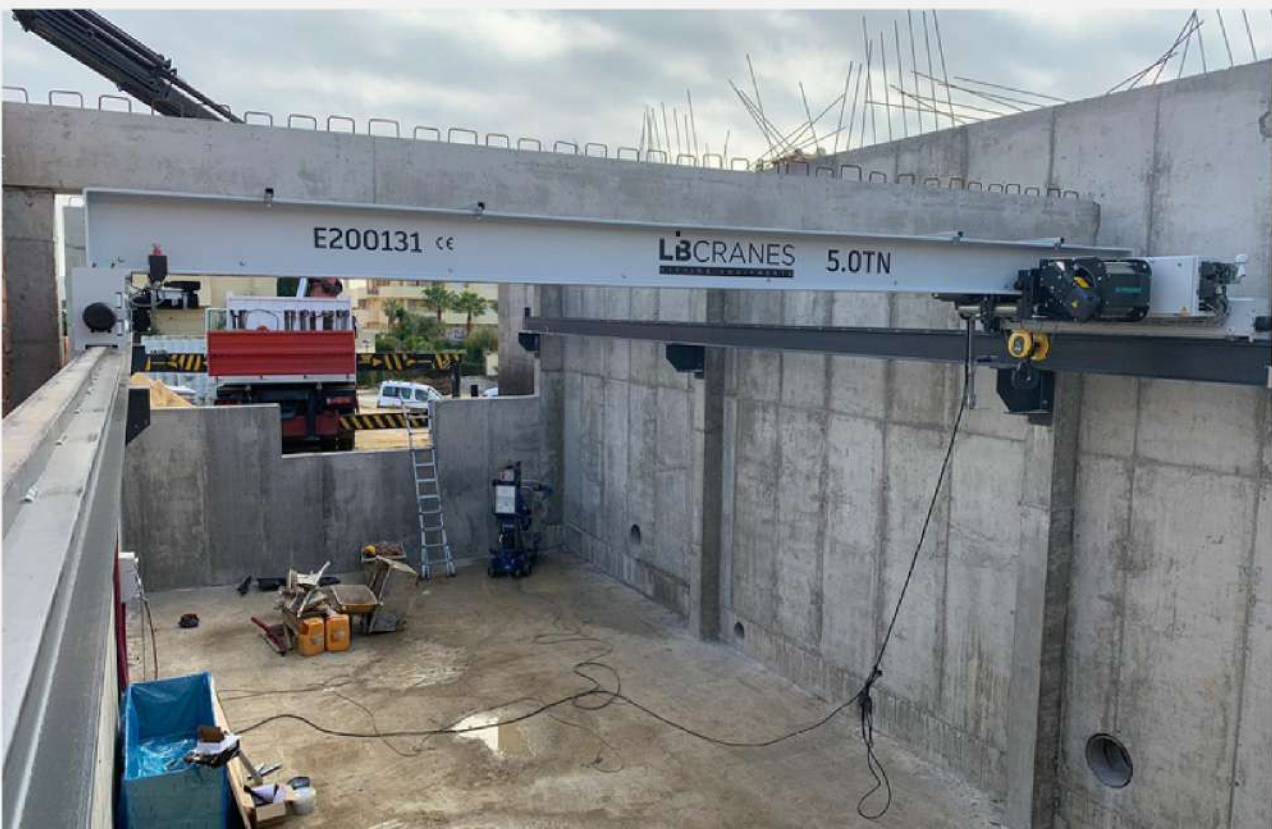
5Tn monorail overhead crane installation
